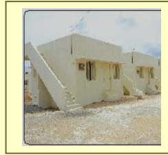
Tsunami Rehabilitation Project 140 Häuser under construction, thereof completed to date 34
